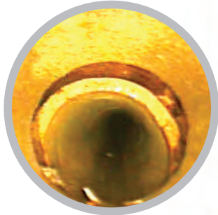
Separated / Offset Pipe
