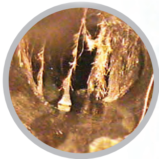
Tree Roots Filling Pipe
