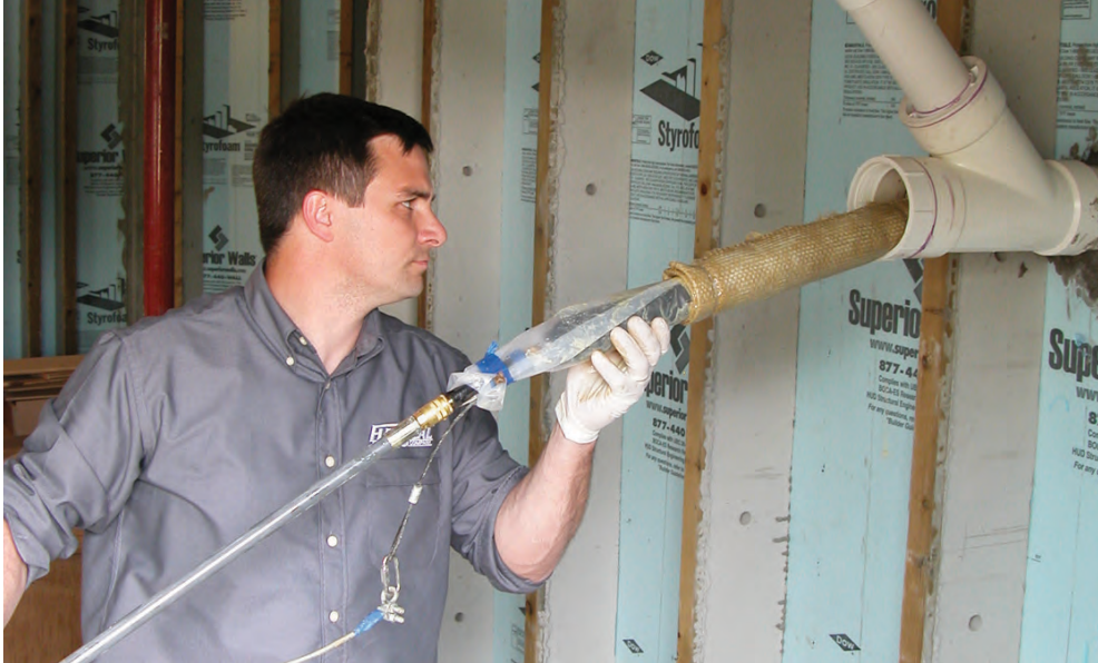
PipePatch conforms to the fitting's exact shape.
