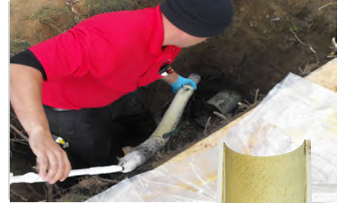
PipePatch conforms to the fitting's exact shape.
